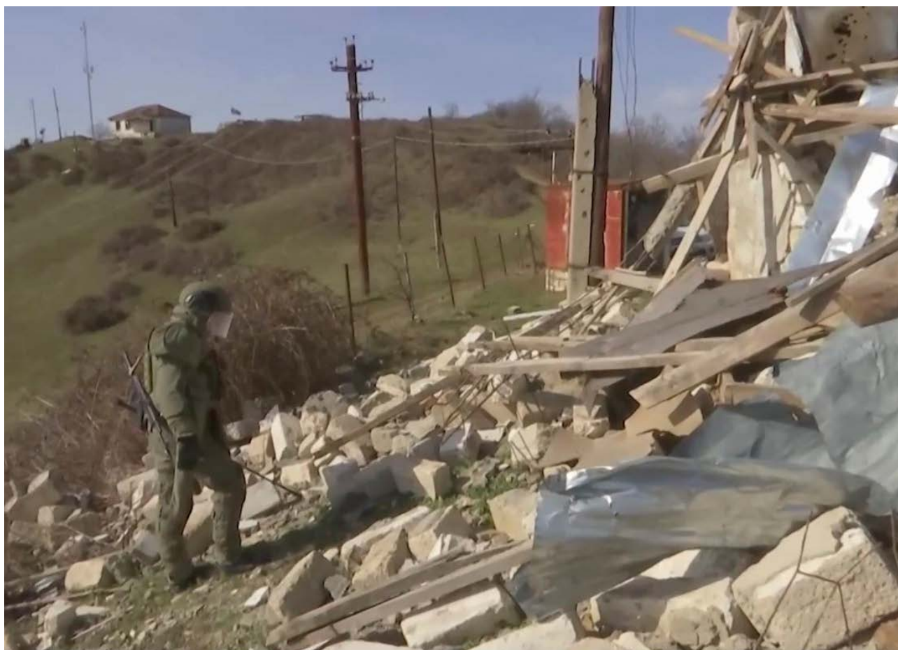
Damage from conflict in Martuni, Nagorno-Karabakh. Photo: Ministry of Defence of the Russian Federation. (CC-BY-4.0).
