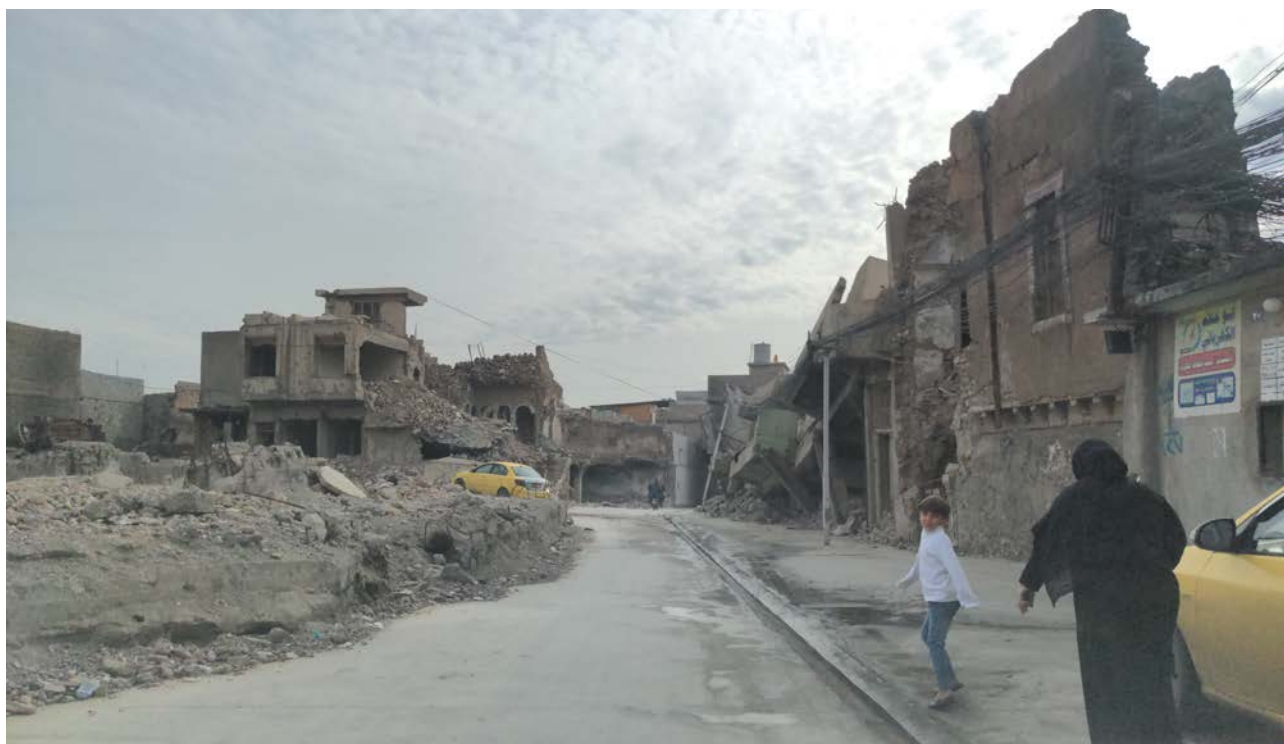
Airstrike damage in Mosul, Iraq, December 2021. Photo: Lonni Friedman (CC BY-NC 2.0)
